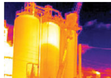
Figure 7 : Level comparison of two tanks
