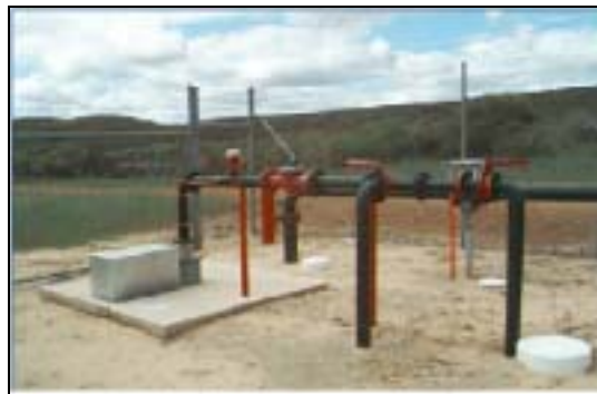
Fig 2 A Typical Bore site at Jurien Bay
